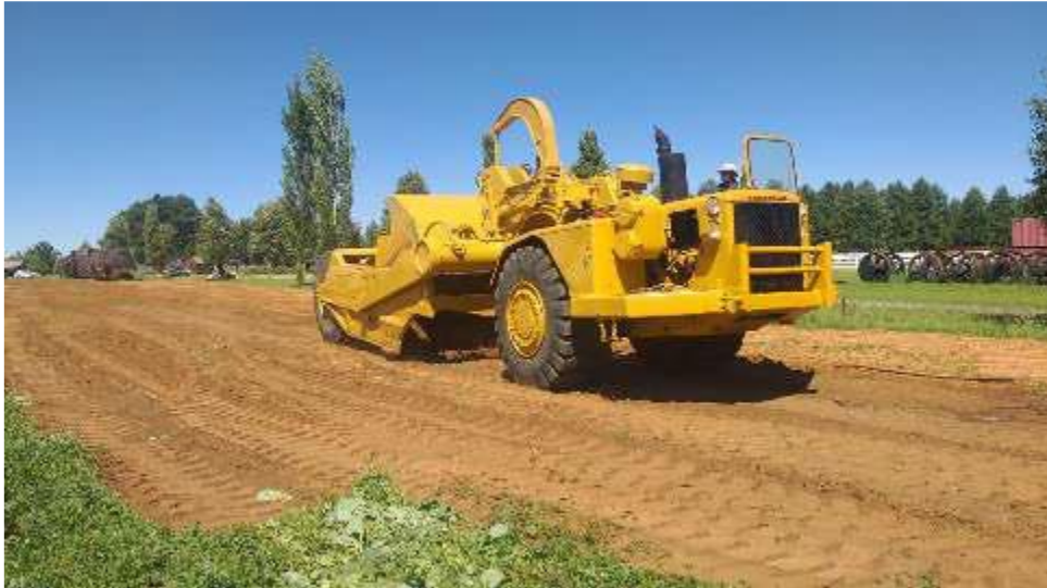
Sandstone's 1965 Caterpillar Scraper prepares the ground for the new arrivals. Picture by Sandstone Heritage Trust.
