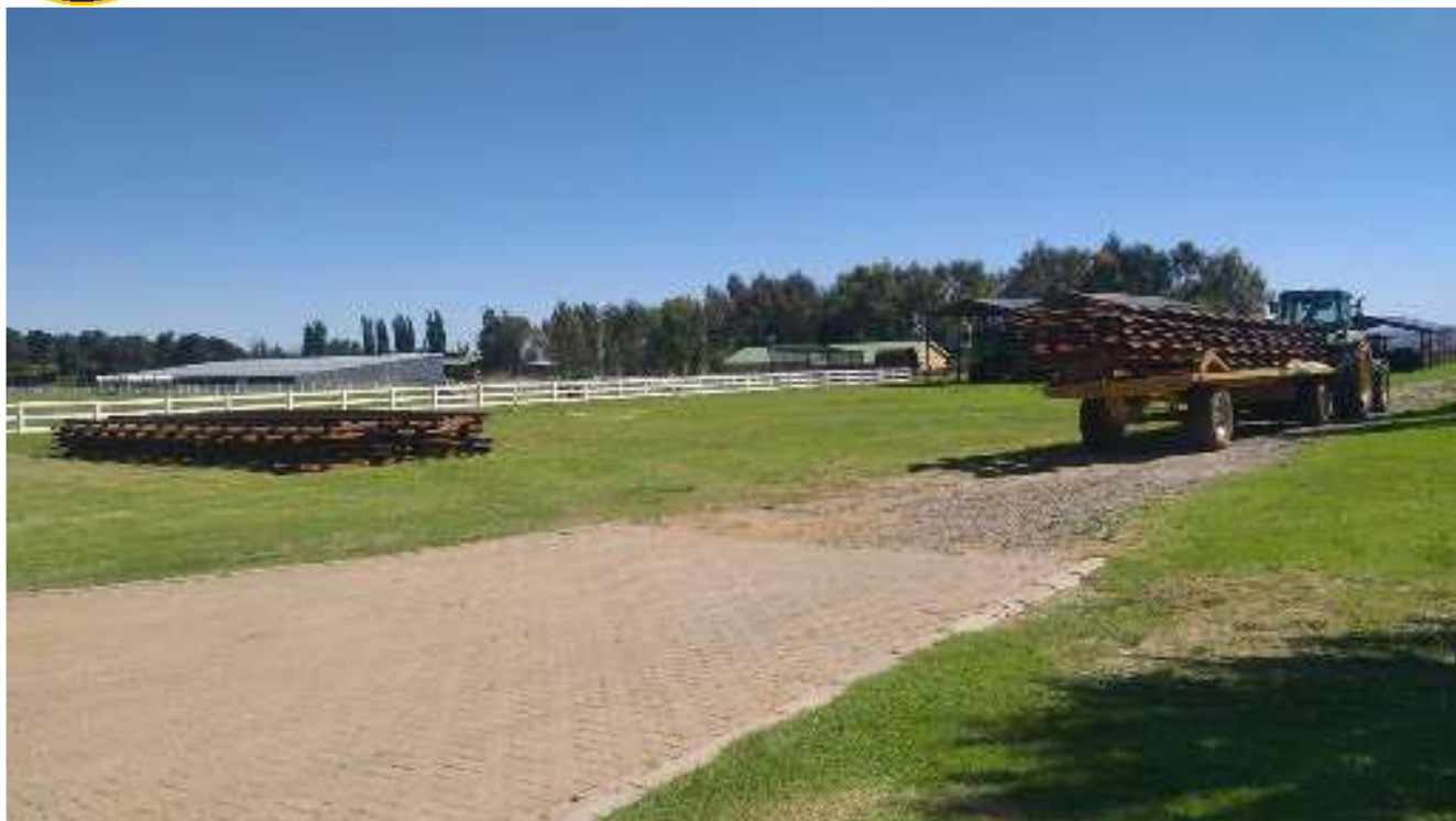
Newly fabricated 3' 6" gauge track panels are brought on to the display site for the impending arrivals. Picture by Sandstone Heritage Trust.
